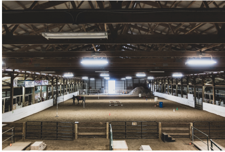
Figure 1: PALS - playground & facility
