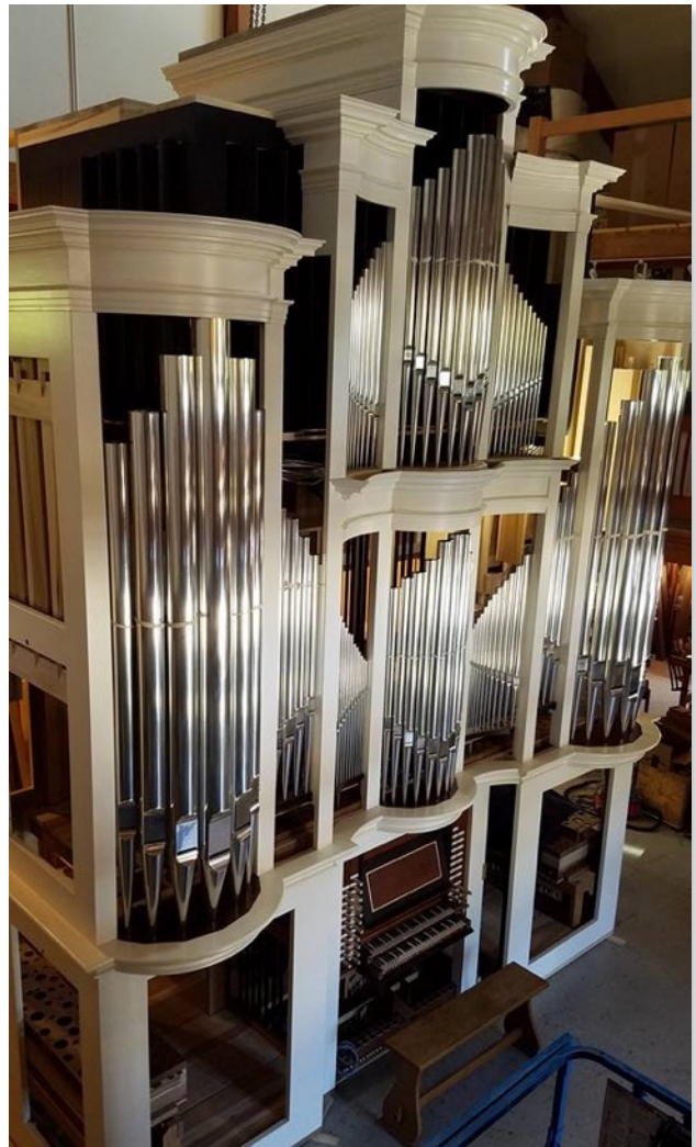
The new Paul Fritts organ (under construction) that is set to arrive at First Presbyterian Church on October 22 Photo Credit: Chris Young
