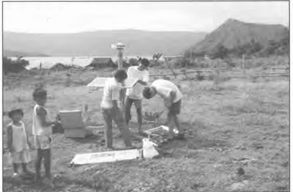
Michael Hamburger works with colleagues from the Philippine Institute of Volcanology and Seismology to install a new GPS volcano monitoring system at Taal Volcano, Philippines.
