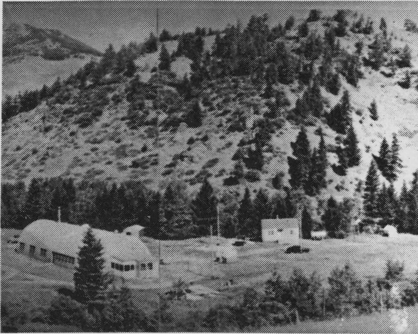
Fig. 4. Upper campus, I.U. Geologic Field Station, 1949. L-R: Lodge, office, tent, resident manager's house, tent.
