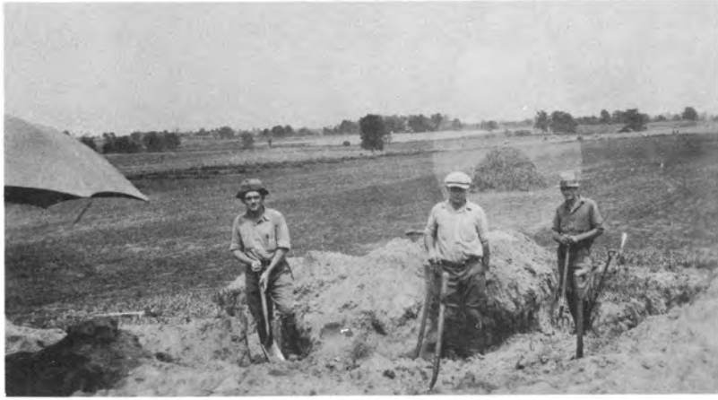
Indiana Geological Survey, Worthington, Ind., 1927. Whitlatch, Kasserman, and Rankin at the shovels.
