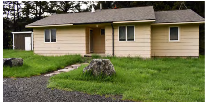
The newly remodeled Resident Manager's house.
